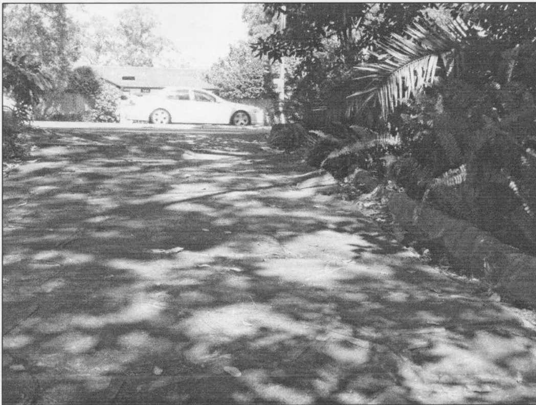
Figure 8 View of fall of existing drive. There is plenty of space for the concrete slab to bridge the root buttress
