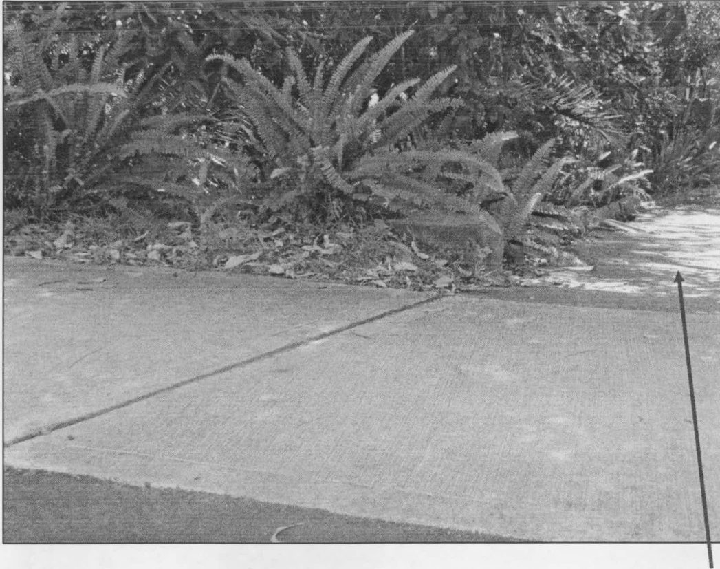
Figure 9 View from the road of footpath and crossover and then the existing drive dropping off to the north
