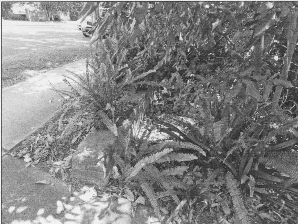
Figure 4 Showing the existing front fence. There are 5 rows of bricks to ground level inside fence and grass clippings
